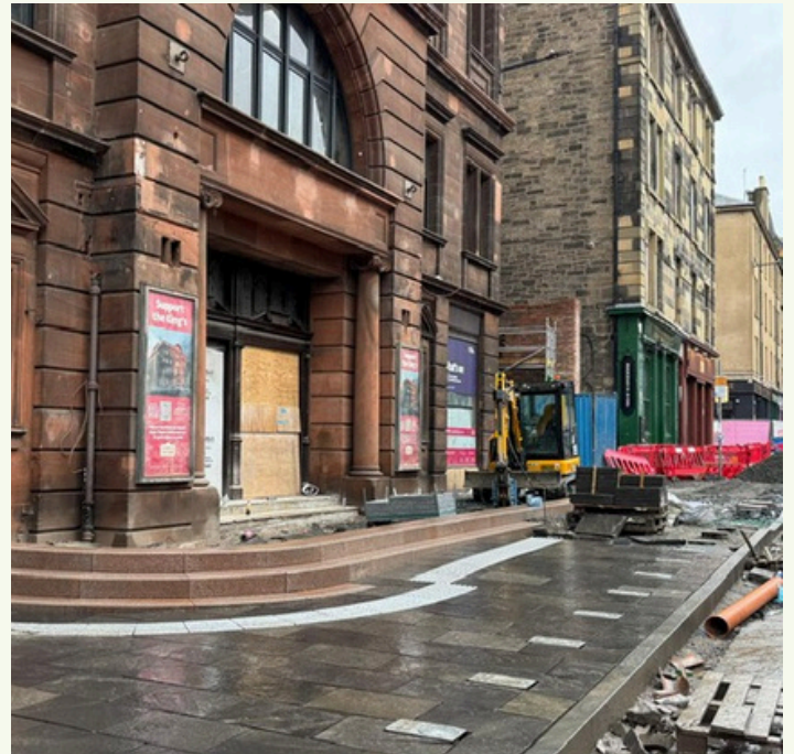
Creating a new level-access into the main foyer. © John Robb
